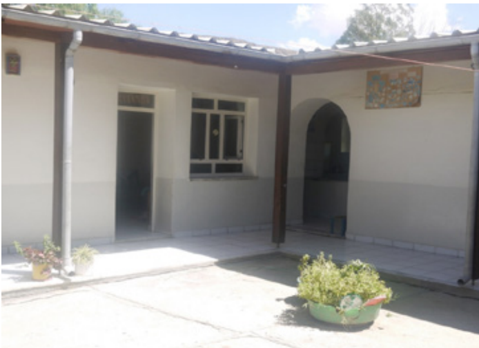
Renovated outside area
